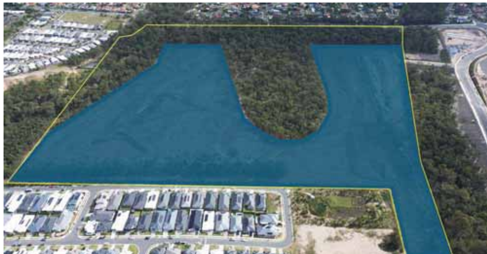
The 28ha site at 257-341 Green Road, Heritage Park, will soon become a 300-home land-lease community
